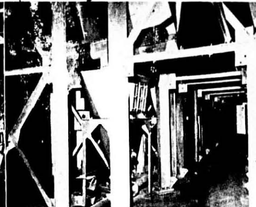
Fig. 9. Lower section of silo installation. Silos feed into vacuum lines (2 lines each serving 10 bins) for delivery to process bins. Silos are paired off, each pair feeding into a common hopper which empties into the vacuum lines. Entire reclaiming operation is remotely-controlled from panel.
