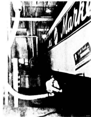
Fig. 1. Truck load of bulk sugar being unloaded at new American Stores bakery in Philadelphia, Pa. in. Attendant connects tube with truck hopper outlet and Fuller pneumatic handling system delivers sugar to storage or processing bins.
